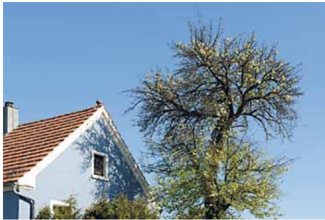
In legal terms, nuisance can be something as simple as branches contacting a roof and abrading the surface.
