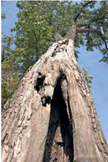
Simply because a tree has a cavity does not mean it will automatically fail soon. The cavity may or may not have structural significance.
