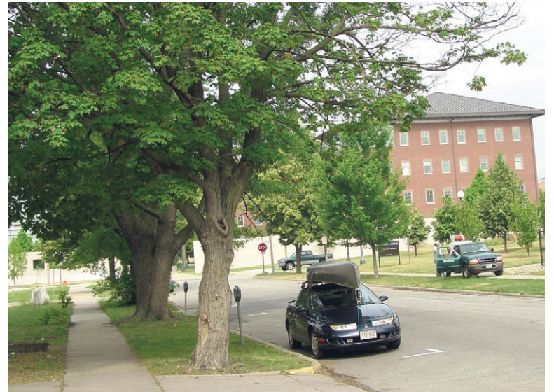
Tree roots can exacerbate the problem of building damage caused by soil moisture changes, since trees are soaking up water through the roots.
